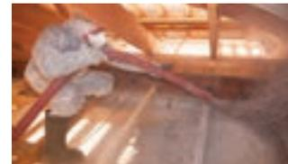
**Blown-in** Also called loose fill insulation, this is a great solution for insulating attics, tight spaces or topping up an existing layer of insulation. Installation is not difficult but it is dusty, sweaty work for two people and you'll need to rent a blower machine. Talk to our Insulation Specialists for availability.
