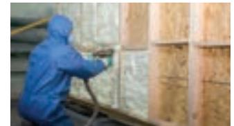
**Spray foam** A very effective insulation when installed properly. It combines 2 chemicals on site to create an expanding foam which is sprayed between framing. It requires special handling, careful application and essential safety precautions. Not recommended as a DIY project, best left to the professionals to install.
