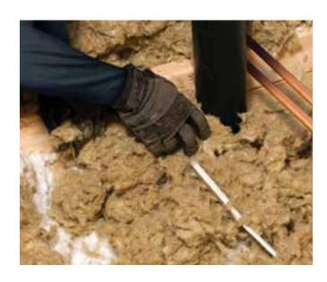
Gaps and voids in the attic can account for up to 30% of the heat loss. Areas around pipe, wiring and attic vents are often neglected and can account for the majority of those gaps and voids. ROXUL ROCKFILL™ loose fill, top up attic insulation makes it easy because unlike other attic insulation, there is no blowing machine required, and installation can be done by hand.
