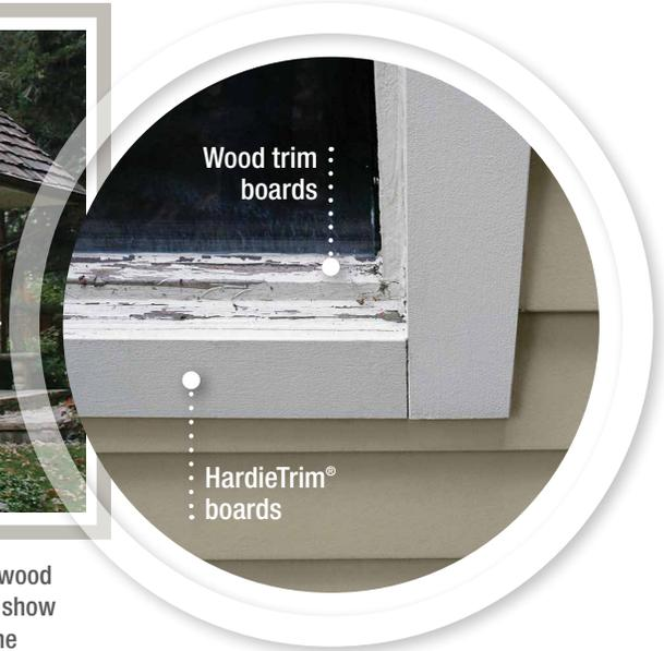
As part of a 2004 re-siding project on a suburban Chicago home, HardieTrim® boards and wood trim boards were all installed and painted at the same time. Today, the HardieTrim boards show no signs of aging, while expansion and contraction have caused cracking and peeling in the wood trim's finish.
